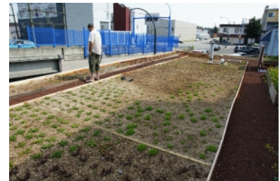
A green roof on the Frog File building, one of two eco-industrial projects built by Toby Barazzuol in downtown Vancouver. Green roofs support green buildings, which is one objective of pursuing eco-industrial activity.
